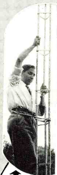
ASSEMBLY GUIDE! Fitting just one leg into pilot hole automatically aligns both sections.
